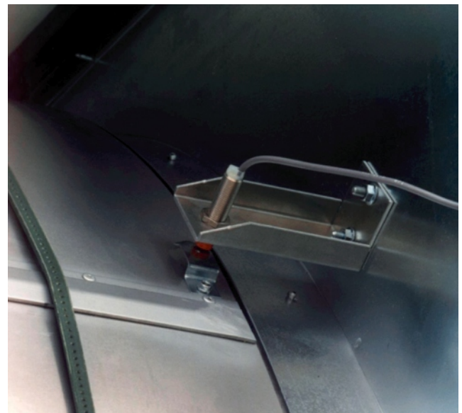
Sensor for rotor operation control
