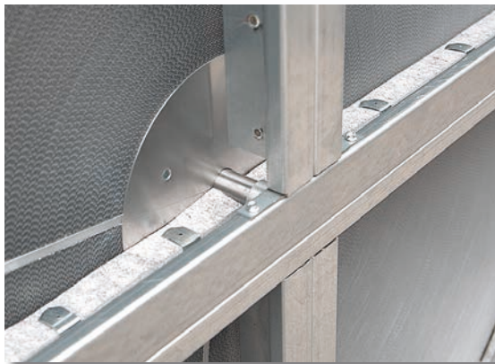
Pressure-stable felt seal for standard ventilation and air-conditioning
