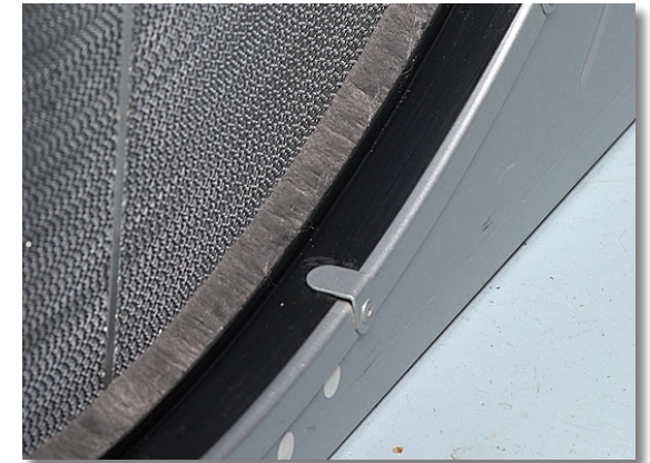
Brush seal for standard ventilation and air-conditioning
